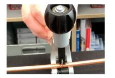
Cut the tube using the tube cutters, being careful not to squash the tube
