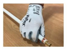
Add a crimp ring and coupler to one end of the pipe
