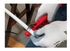
Measure and cut the PEX pipe at 7.5ft or 90 inches
