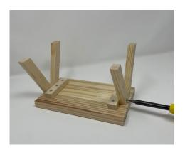
**Step 2:** Install all 4 legs (C) using screws into pre-drilled holes securing to the tabletop brace
